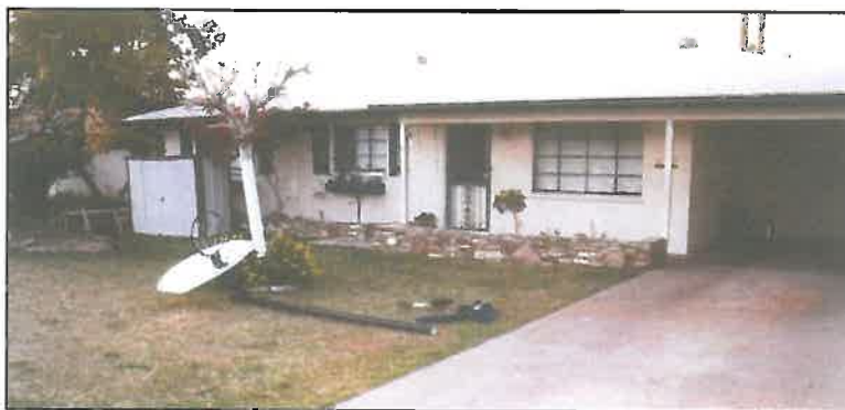
Photo 1a 2 . Broken pole in yard.
